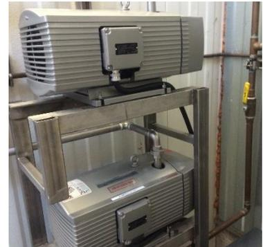
Figure 3: Electric vacuum pumps installed to replace compressed air.
